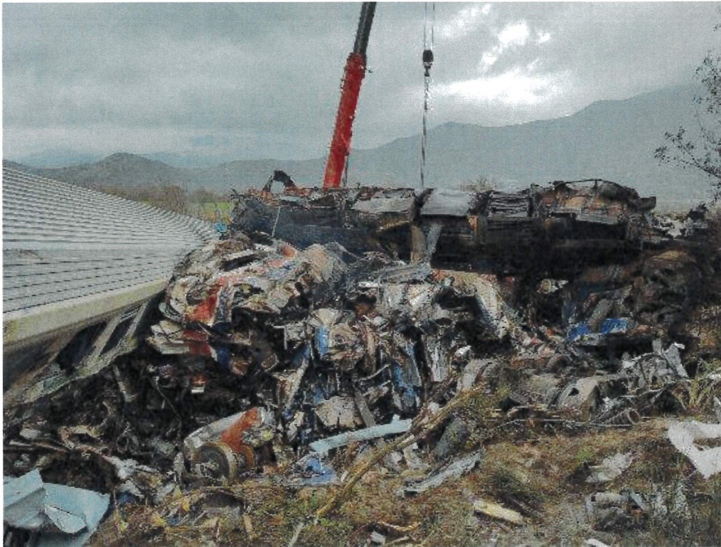
Figure 21: wreckage around transformer and fireplace - file: 230301_073502.jpg
