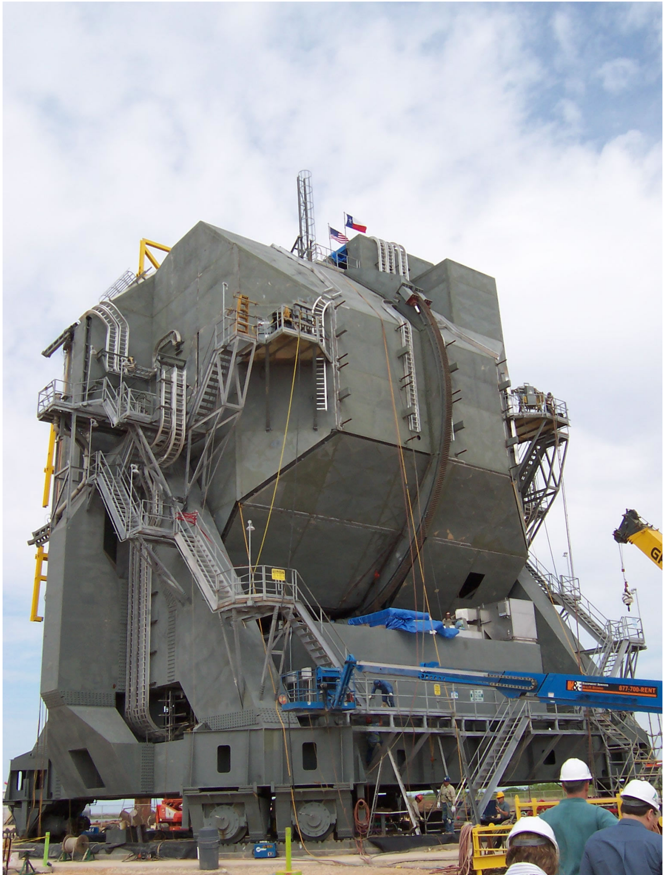
SBX radar mount at Ingleside
