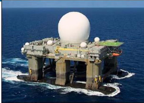
SBX-1 Platform during sea trials in the Gulf of Mexico
