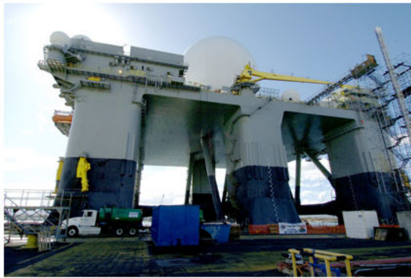
The X-Band radar platform is large enough to accommodate 18 basketball courts on its six pillar legs.
